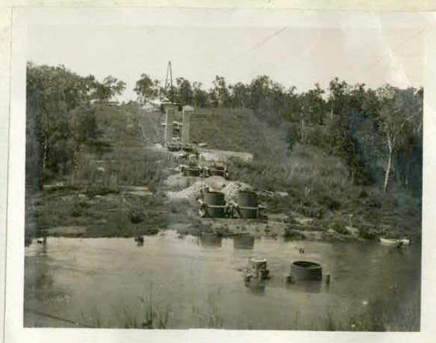
Bridge over Katherine under construction
