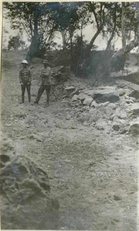
King River Crossing Before improvement.
