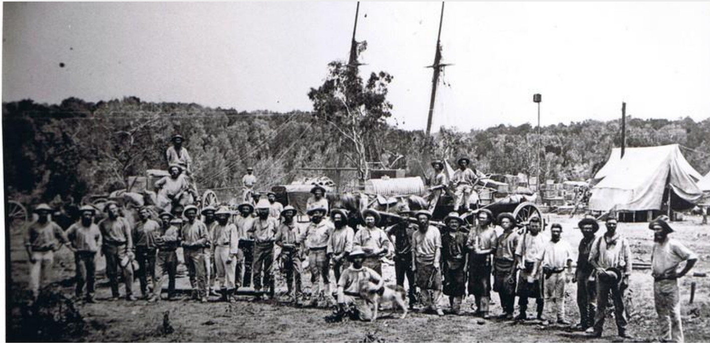
Roper River Jetty
